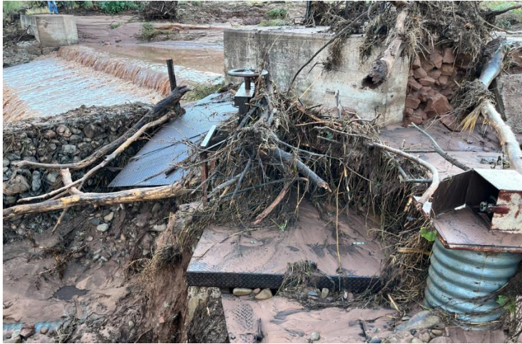
(The picture shows the Ditch 2 sandbox with heavy metal plates ripped off the top.)
