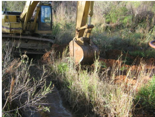
A track hoe was used to clean the area above the dam
