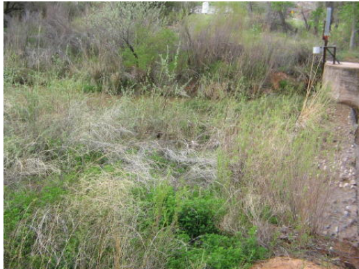
North Ditch One Head Gate
